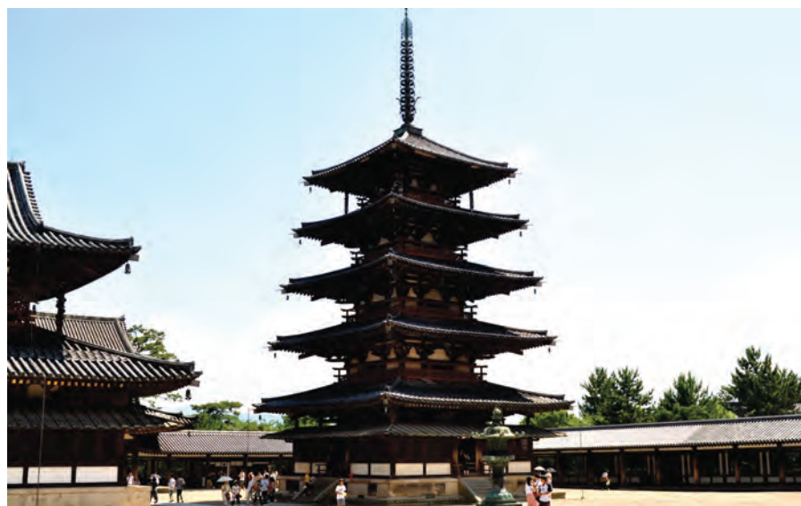
Fig. 1 – The five-story pagoda on the grounds of the historic Horyuji Temple in Nara, Japan, is among the oldest wooden structures in existence, dating back more than 1300 years. The resilience of this ancient building lies in the material from which it is constructed, a type of cypress with a natural defense system that repels insects, withstands toxins, and keeps harmful bacteria and fungi in check. Courtesy of Urabe Research Laboratory, Japan, www.uraken.net .
