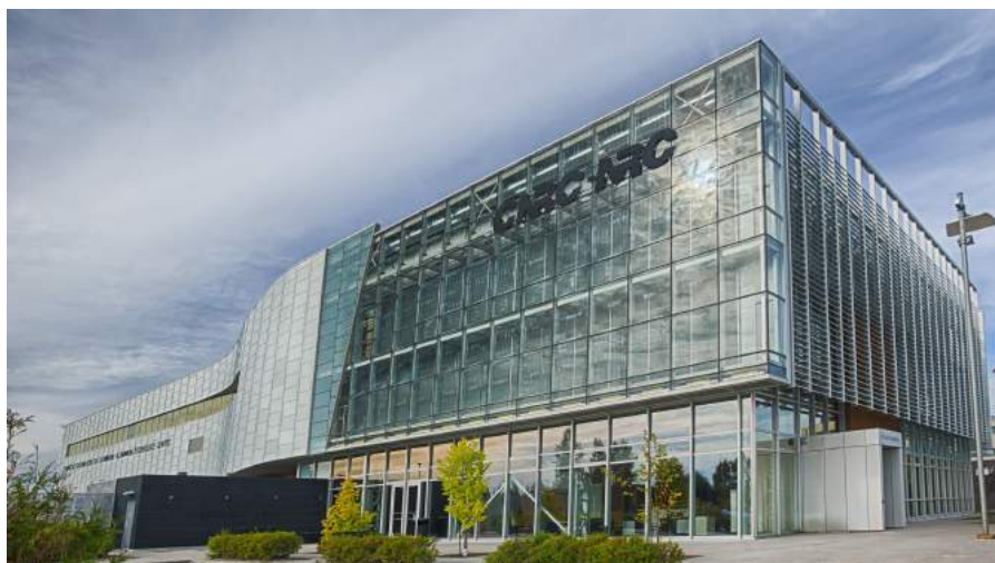
The Aluminium Technology Centre in Saguenay, Quebec, Canada.
