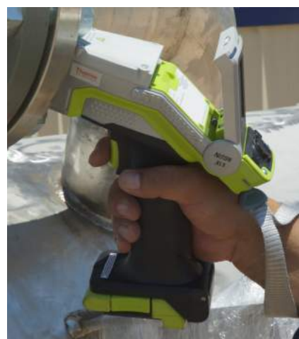
Thermo Scientific Niton XL5 XRF analyzer inspects finished welds in steel piping.
