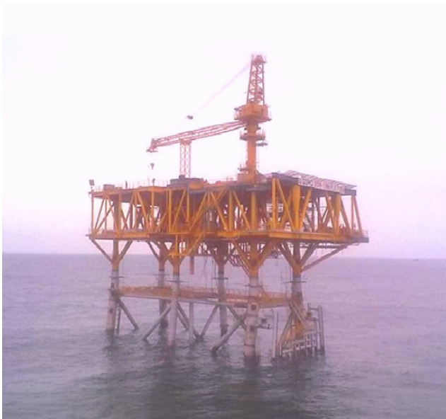
Fig. 7 — TSAC applied on splash zone of installed offshore platform.
