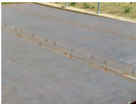
Fig. 4 — HiDep weld—two 8 × 20 ft steel plates.
