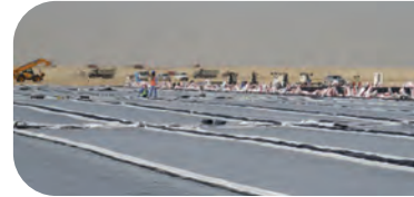
A new material, being installed at a site in the Middle East, combines sodium bentonite clay and polymers to create a substance that can withstand industrial waste. Courtesy of CETCO.
