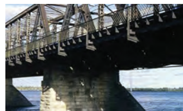
Victoria Truss Bridge, built in 1898. Courtesy of Hugh McQueen.
