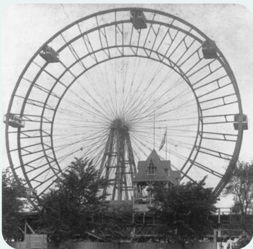
The first use of alloy steel in the U.S. was for the axle of the famous Ferris Wheel at the 1893 Chicago World's Fair. Courtesy of Library of Congress.
