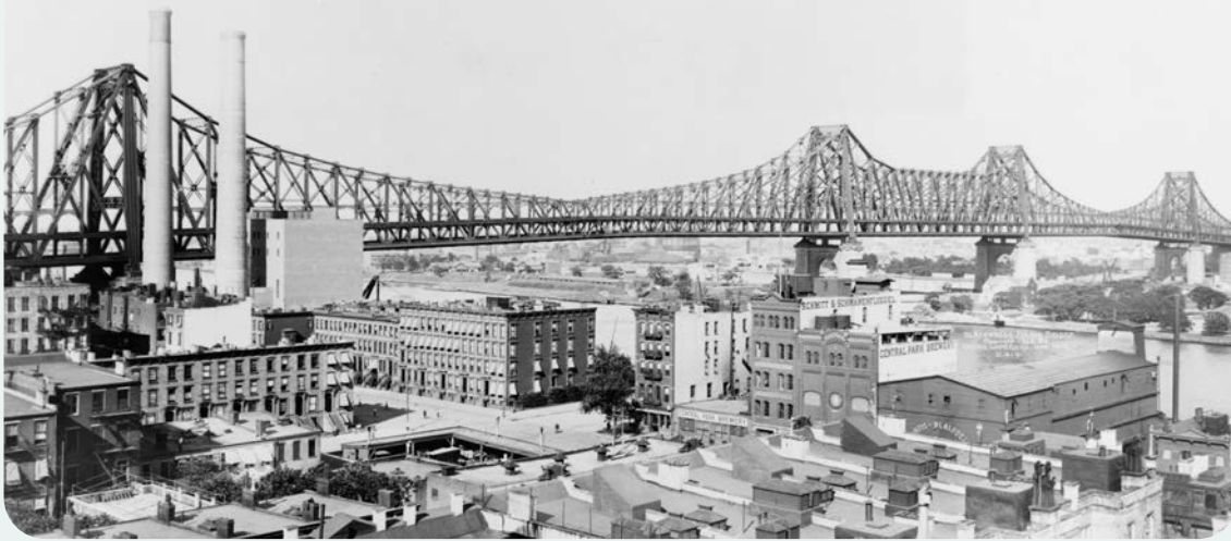
Queensboro Bridge made of nickel steel, New York City, circa 1908. Courtesy of Library of Congress.
